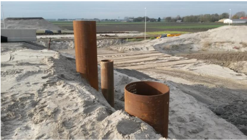
Figure 2.9: Overview of the steel piles.
