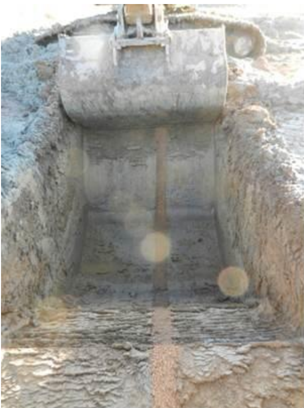
Figure 2.3. Visual inspection of an in-situ vertical underground screen of Trisoplast
