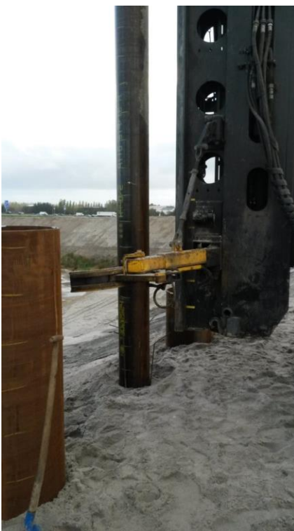
Figure 2.10: Junttan HHK-5a Hydraulic block with steel pipe.
