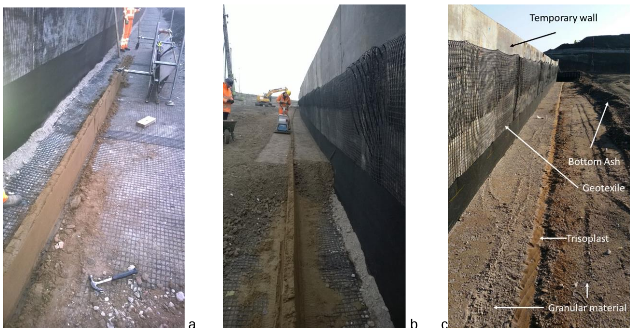
Figure 2.1. The overview of the on-situ installation of a Trisoplast liner
