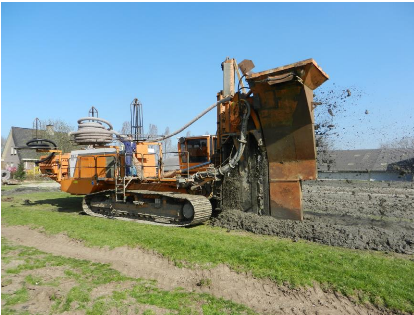
Figure 2.2 In-situ installation of a Trisoplast vertical underground screen
