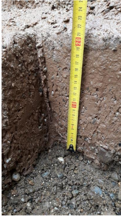
Figure 2.7: excavated underwater installed Trisoplast layer.
