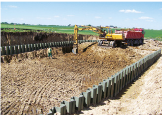
Retention tank by the motorway.
