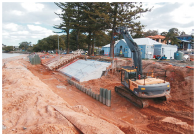
Protection of the seawall.
