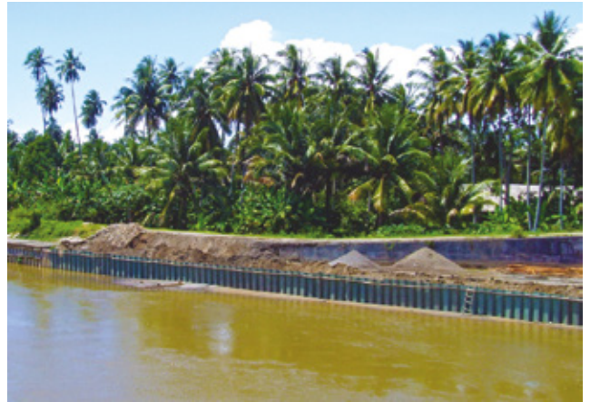
Anti-erosion protection of the river-bed.
