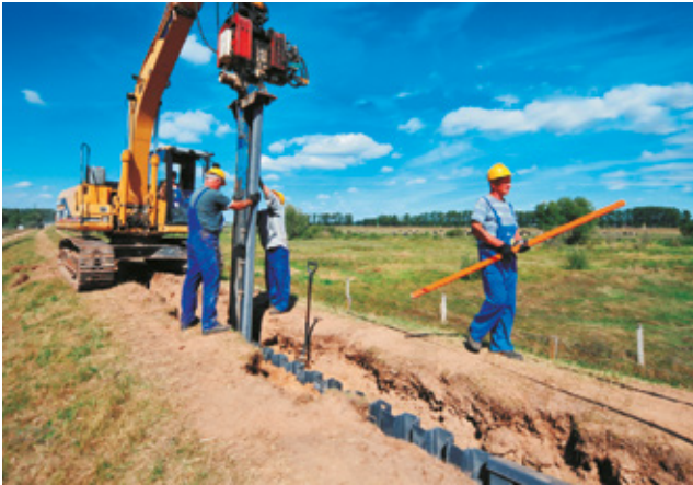
Sealing of the flood embankment.
